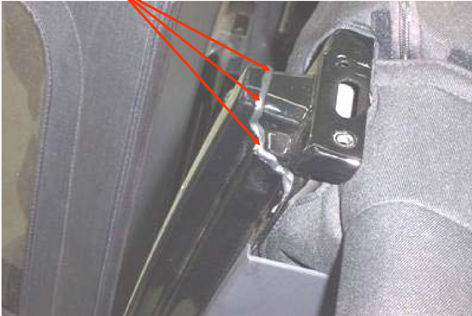
Top of Right B – Pillar With Mocket Seal removed
